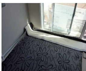
Implantation de la moquette Laying the carpet
